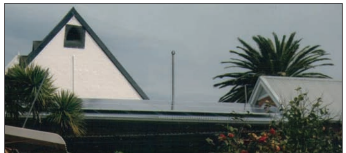
POWER dressing... solar panels atop Leighmoor UC's roof
