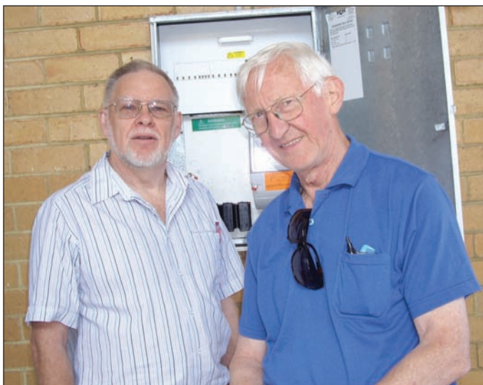
Above: David Evans, friend and solar advisor to Leighmoor and Geoff Serpell, Council Chair, at the newly installed smart meter to conduct power from the panels to the grid.
